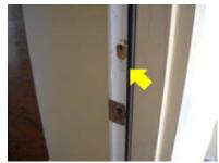
The front door is in need of additional coats of protective finish. Stained doors of this type need periodic maintenance. To properly protect the wood and finish they should be sanded and additional coats of finish applied every few years. It should be verified that the top and bottom edges are also sealed. These type doors often warp when these edges are left unsealed.
