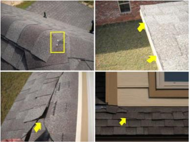
The shingles are in acceptable condition and well within their useful life. I test the condition of the shingles by placing the palm of my hand on the shingle, appling pressure and rotating it. The amount of granules that break free is an indication of the condition of the roof covering. Very few granules broke free from these shingles.
