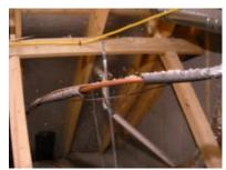
The compressor unit is not sitting level. It should be on a level platform.
