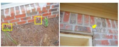
Brick veneer siding is now required to have weep holes (mortar vacancies every few bricks, allowing moisture to escape). Some of the weep holes are below the grading. When below grading, insects may enter the property more readily. At the very least a chemical barrier should be maintained to keep pests out of the home.
