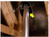
The black foam pipe insulation should not be within 6" of the water heater draft hood. It is a combustible material.
