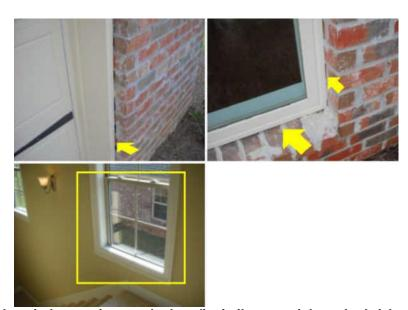
Seal the window casings and other dissimilar materials to the brick.
