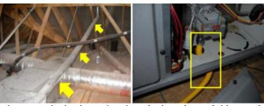
The ratio between the horizontal and vertical portions of this vent is not correct. This can create drafting and condensation problems. I
