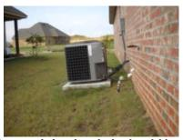
The compressor unit is not sitting level. It should be on a level platform.
